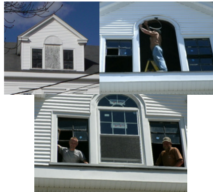
100 Main St., Bar Mills, BHHS Attic Window Replacement Renovation
