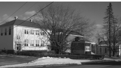
Exterior of 1930 classroom section with attached 1957 gym annex; Buxton Center Baptist Church on right.
