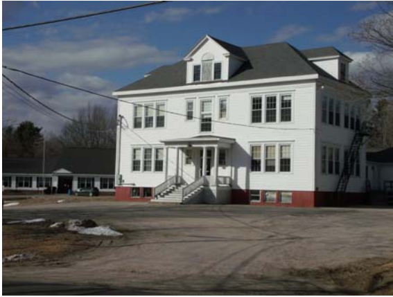
Old Bar Mills Elementary School —a Contributing Building in a DOT National Register Historic District
