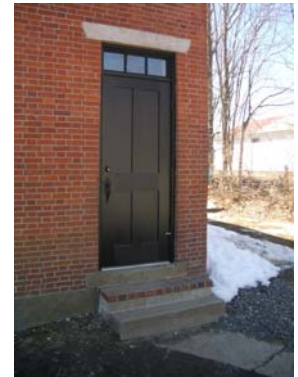
New Door and Transom at Historic Elden Store
